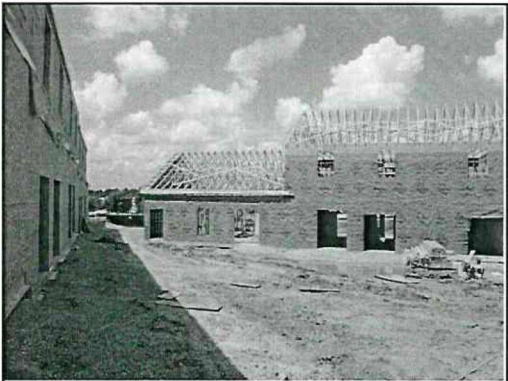
Framing building C
