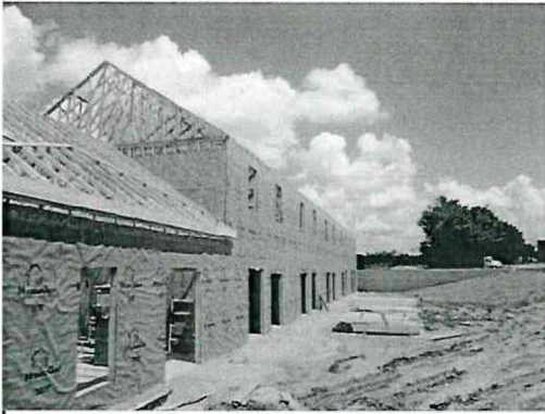
Framing building C
