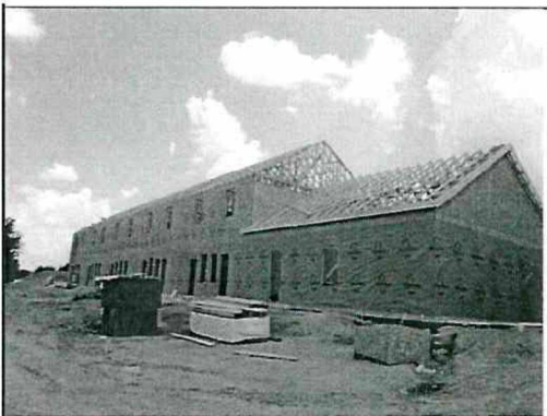
Framing building C
