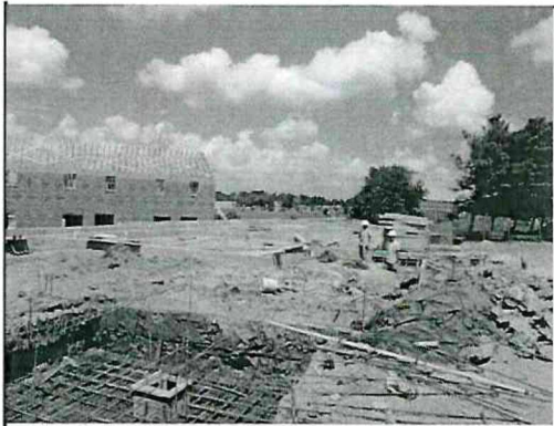
Building A foundation walls and elevator pit
